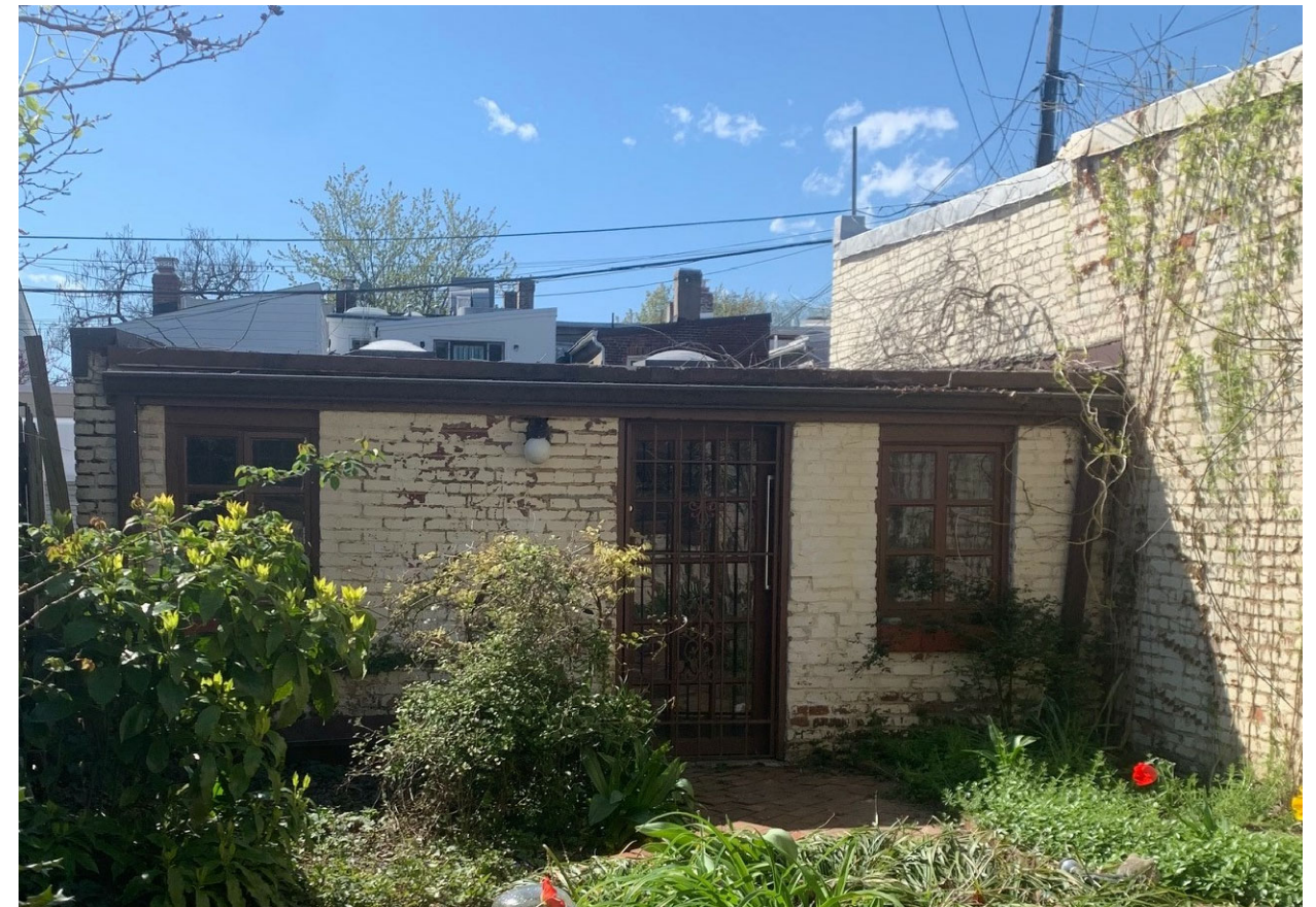
EXISTING GARAGE FROM BACK YARD
